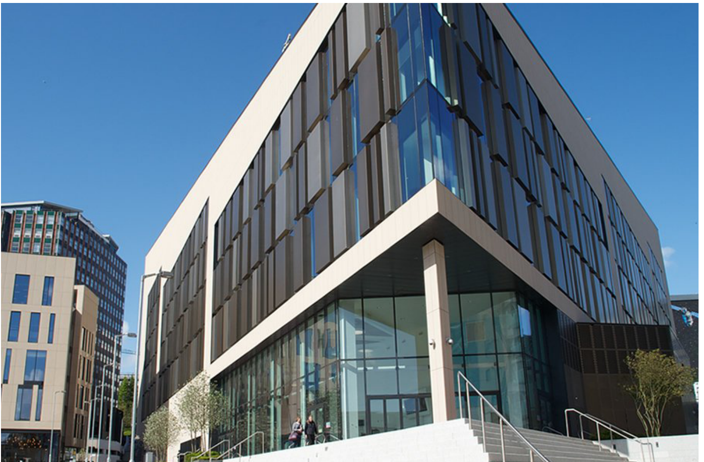
Fig. 4.5: Technology & Innovation Centre at University of Strathclyde.
